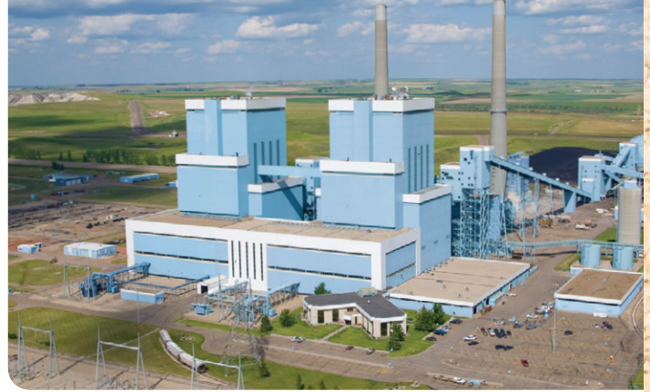
Antelope Valley Station
